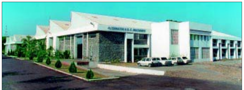
AC Generator Plant
